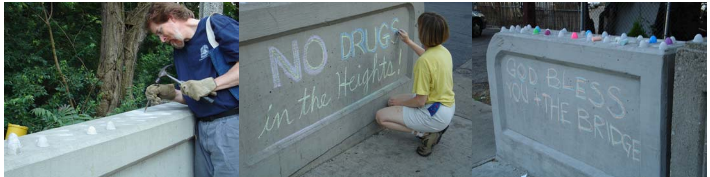
After the Kennedy Heights bridge was prepared for the bump molds, concrete was poured into Easter eggs and attached to the bridge. At the bump party, CPOP members wrote anti-drug messages in chalk.
